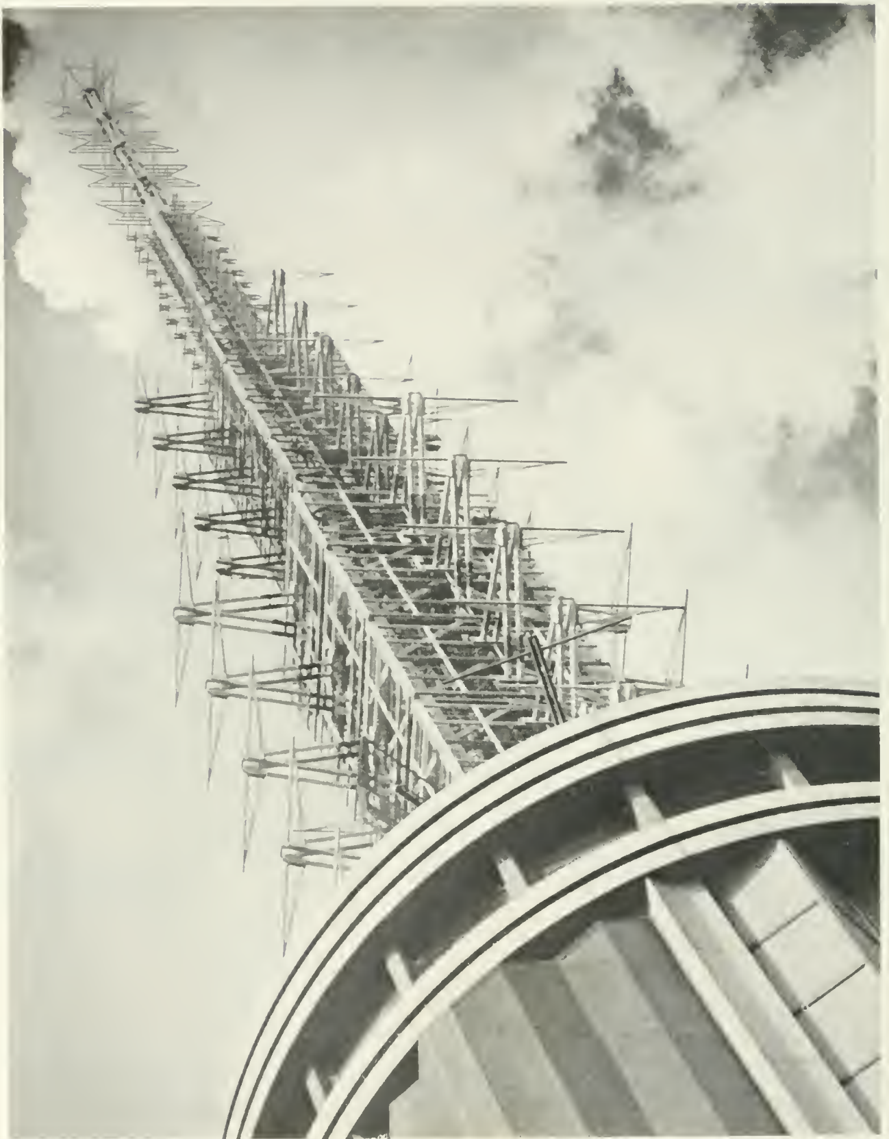
Antennas for five TV and three FM stations are supported by this 200-foot mast atop the Empire State Building. The array was designed by RCA engineers.
